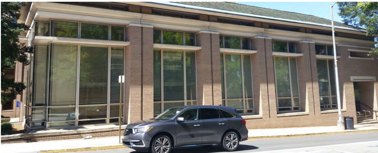
Columns are 2 ft 4" deep
