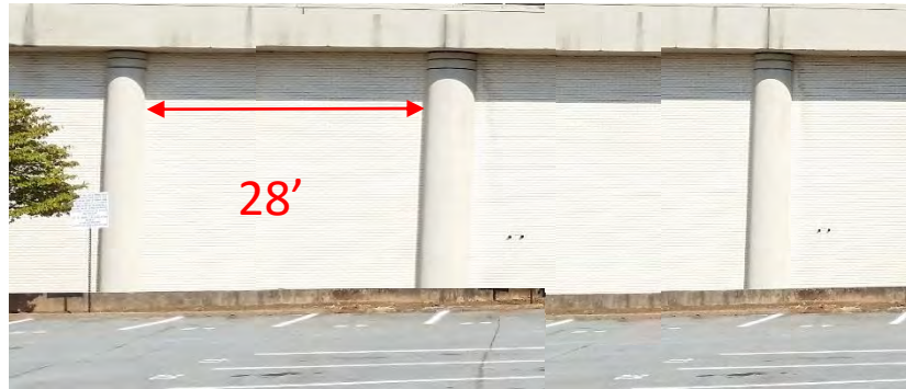
Half columns project 19" from wall plane
