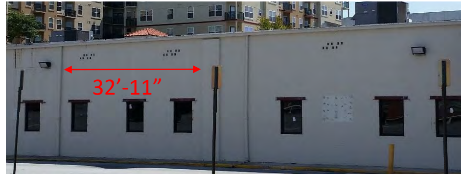
Pilasters project 4" from wall plane
