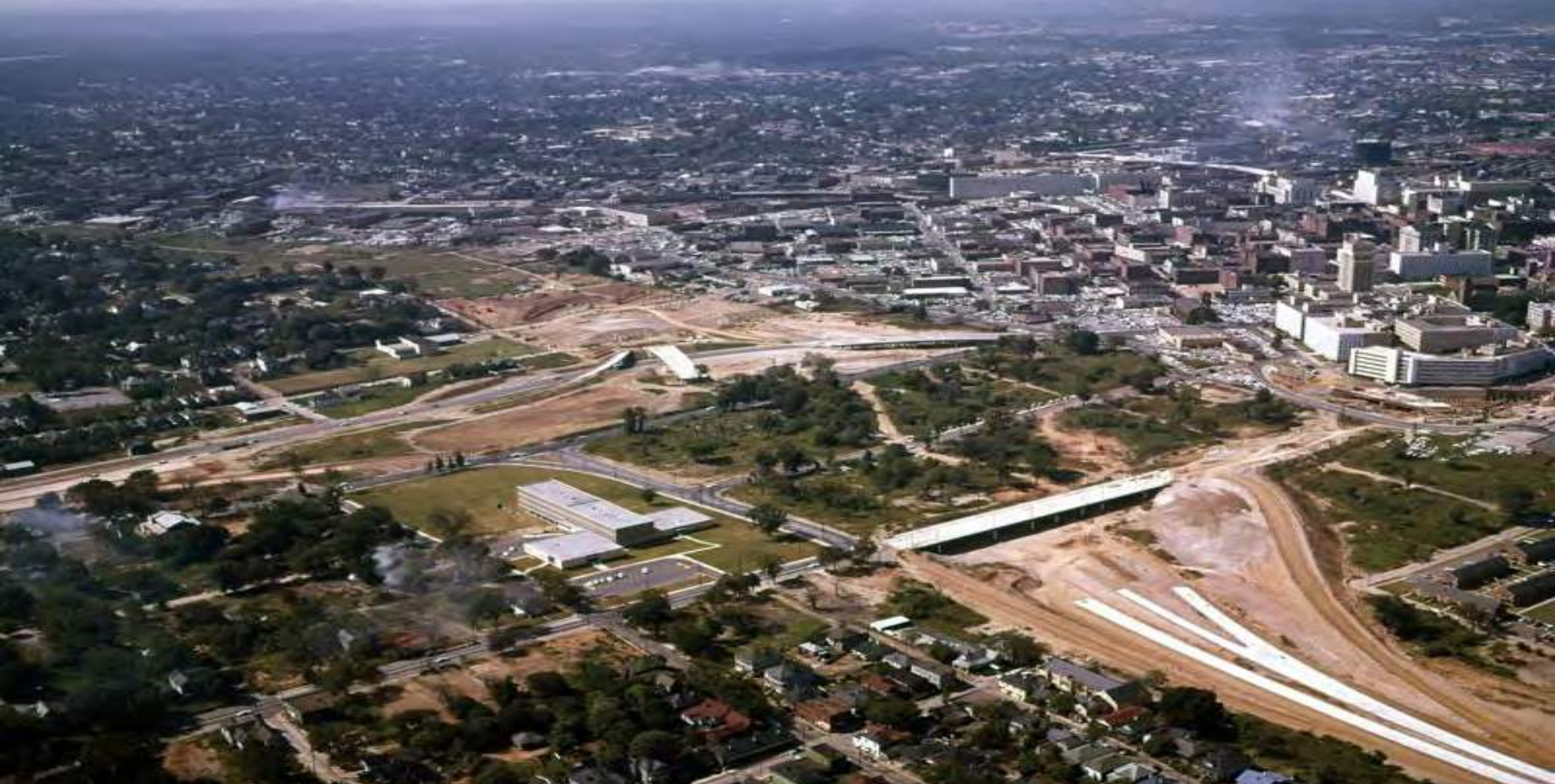
Aerial view over the construction of the Downtown Connector near the Georgia State Capitol building, looking southwest, Atlanta, Georgia, September 27, 1961. Photo: Floyd Jillson/AJC
