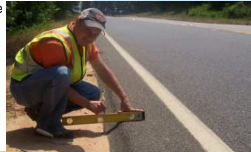
Example of the SafetyEdge SM after backfill material settles or erodes. Source: FHWA
