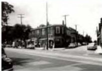
The corner of West Broad Street and Roberts Street, shortly before demolition for the I-16 exit ramp.
