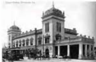
Union Station passenger rail terminal opened for business in 1901 between Roberts and Stewart Streets.
