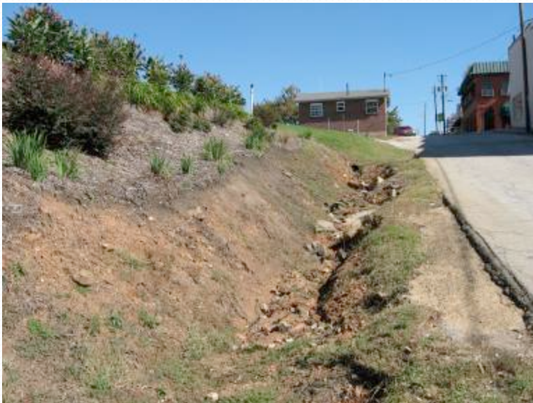
Stormwater problem in downtown Cornelia
