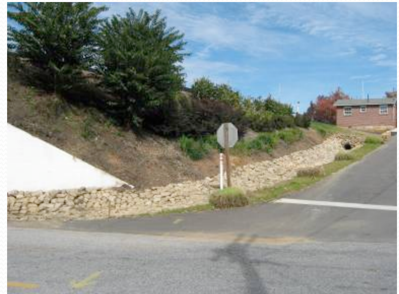
Stormwater problem in downtown Cornelia
