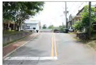
CHOICE STREET: LOOKING SOUTHWEST
