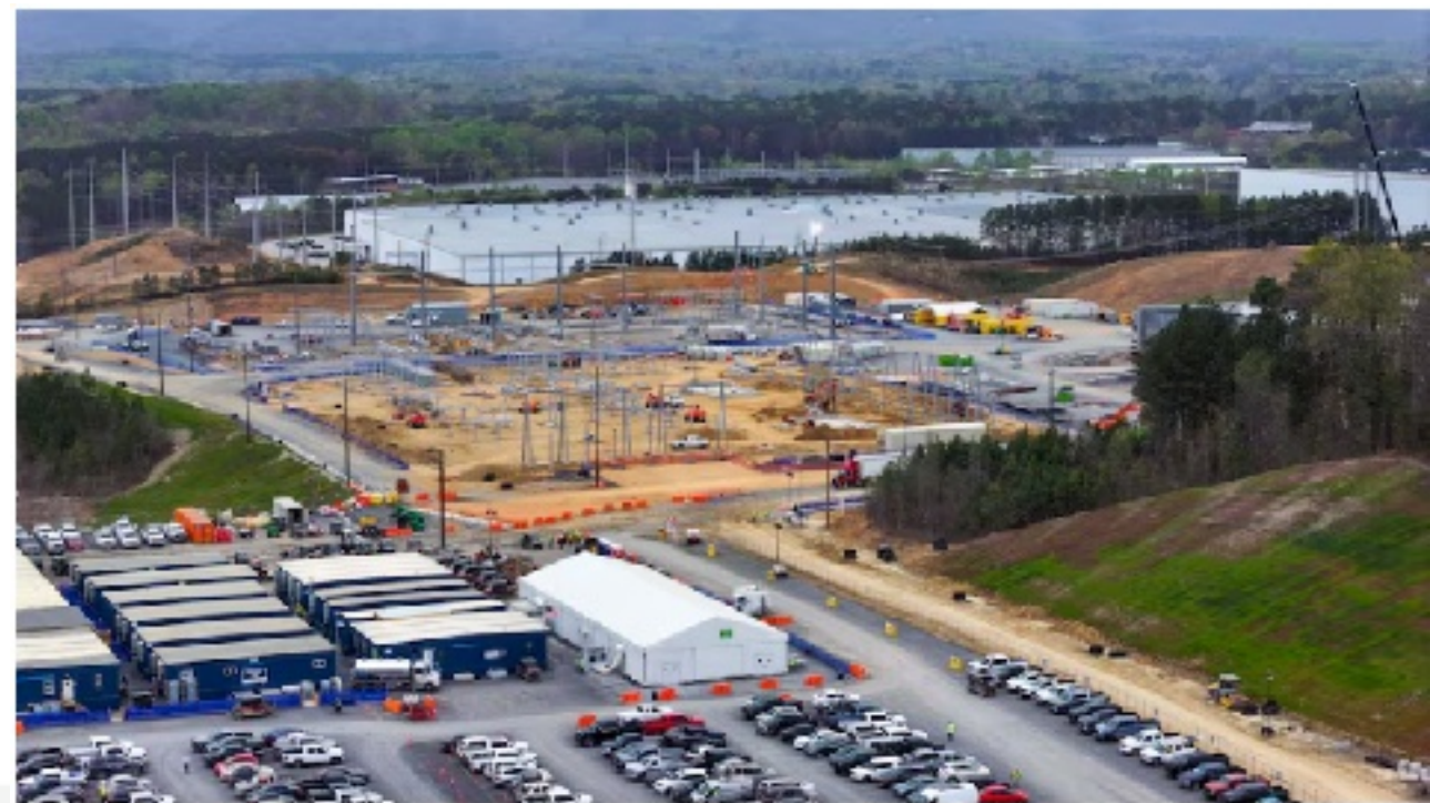
This aerial image shows the 175-acre construction site for Core Scientific, a crypto and AI data center company that has expanded its presence in Dalton. Residents in the nearby areas complain about noise pollution caused by heavy equipment.
