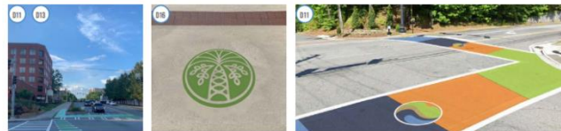
(Left to right) High-visibility bike crossings and painting buffers along multiuse path; Sidewalk decal (National Highway Products); High-visibility crosswalks indicating trail path
